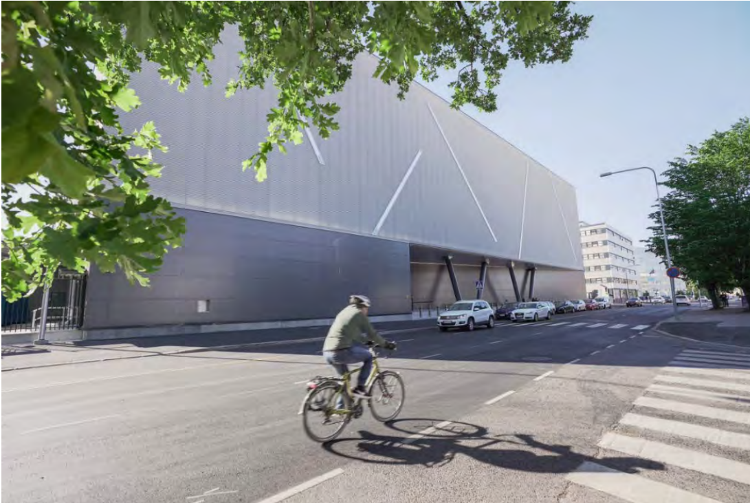
Figure 6. Telia Helsinki Data Center. Copyright Telia.
