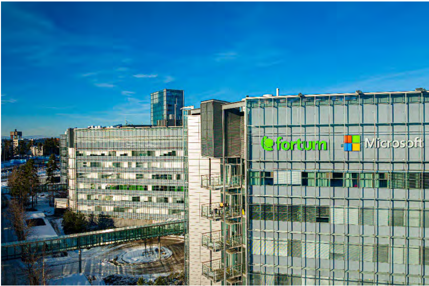
Figure 9. Large-Scale Waste Heat Project by Microsoft and Fortum launched in Espoo. Image: Fortum.
